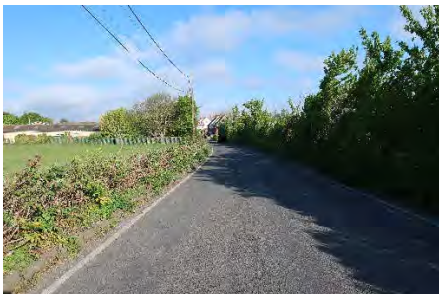
Eastern side – Road alignment.
