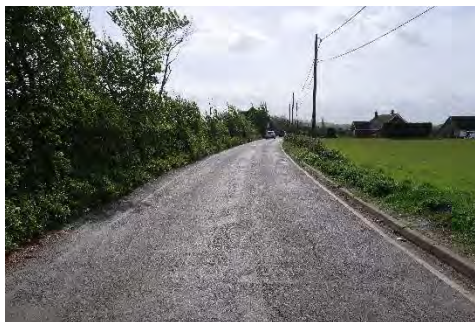
Photo 5 Carriageway edge lines.
